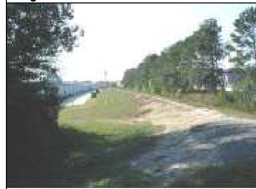
Figure 4.16: Picture of a Slidell LA Levee
