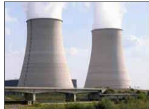
Figure 4.19: HAZMAT Nuclear Facility
