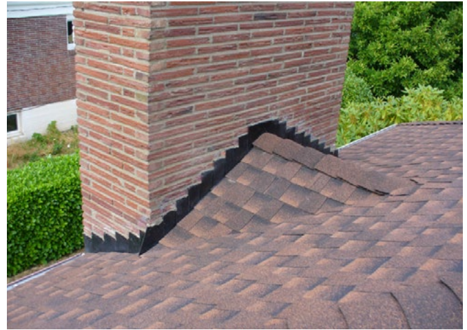
Cricket or saddle at chimney.
